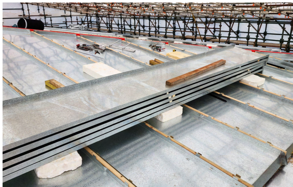
Replacement of the Senate Chamber roof following damage from the 2020 hailstorm; Photos: Daryl Leishman.
